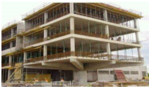
Figure 2: (A) Floating column used on Structure in construction, (B) Palestra in London, United Kingdom
